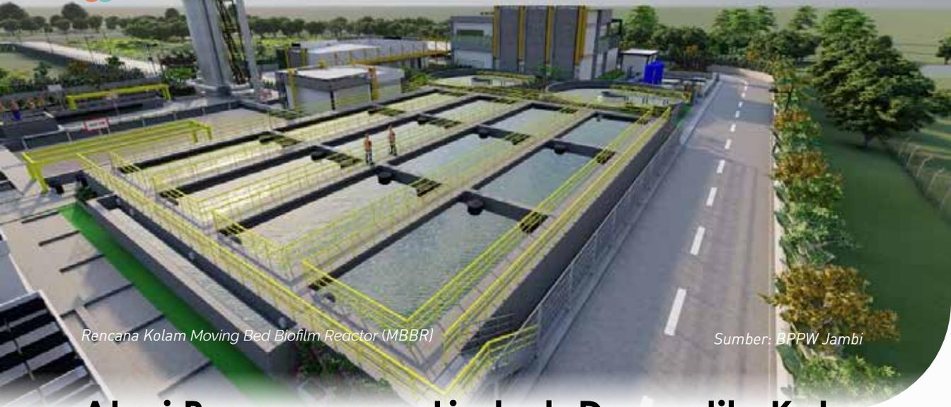
Rencana Kolam Moving Bed Biofilm Reactor (MBBR)
